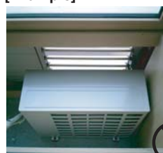
<Without air guide> Safety device activation
